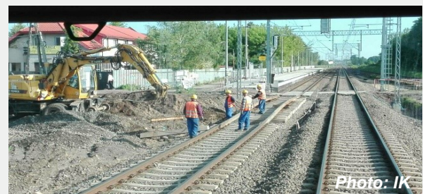
Photo 1. Works on the railway line no 8
