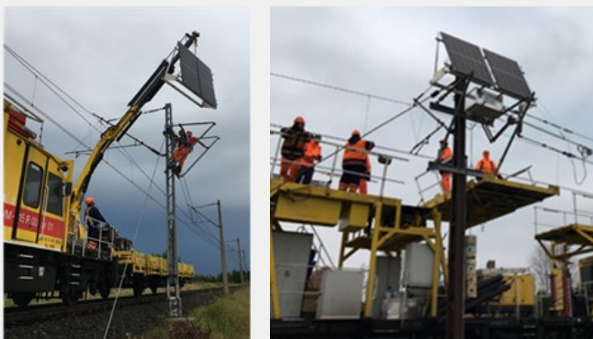
Fig. 1. Installation of the anti-theft system on the IK test track
