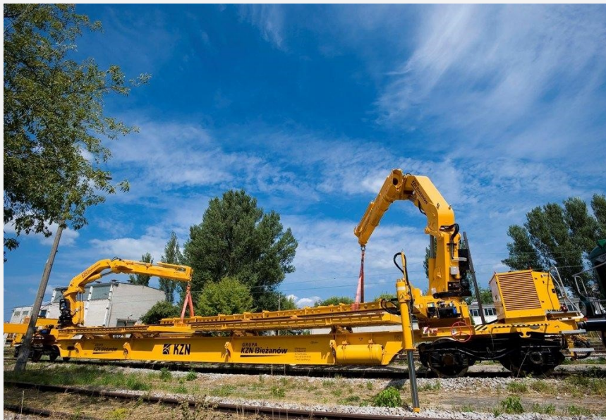
Photo 3. Loading of the wagon with a secured turnout using HDS cranes
